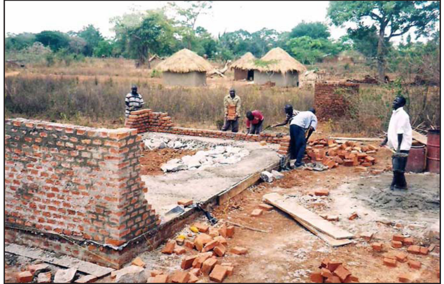
Construction underway. Photo by community member
